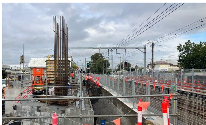
Above: Lift shaft, footbridge and platform works.
