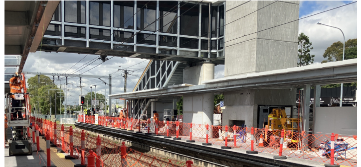
Above: Platform works during a scheduled track closure.
