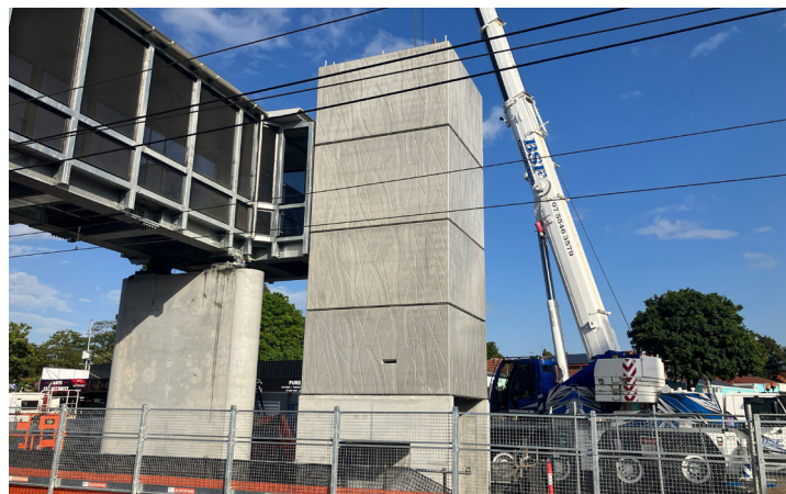
Above: Installation of new footbridge and lift shafts.
