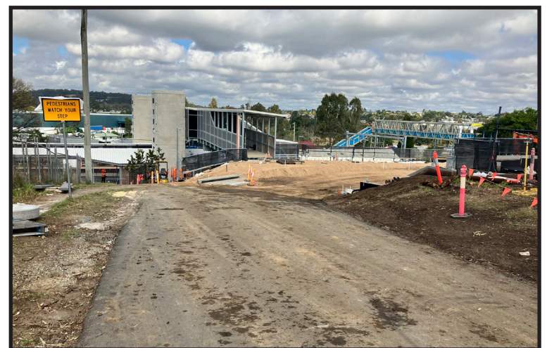
Works for new entry ramps, carpark and kiss 'n' ride area
