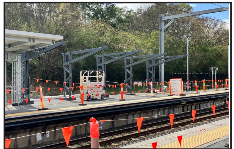
Platform shelter works on new, fully raised platform
