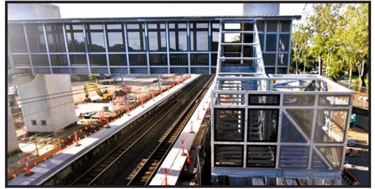
Platform raising, lift and footbridge works (above)
