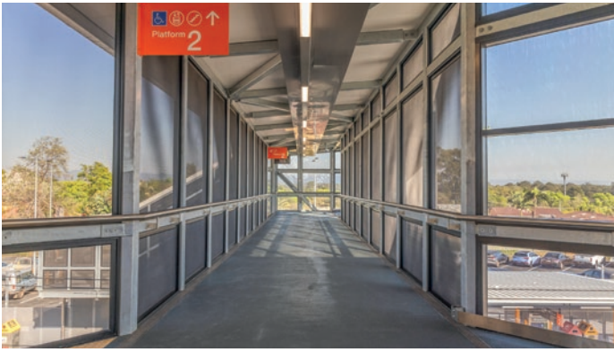
Footbridge with lift, ramp and stair access
