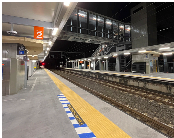
Above: Upgraded platforms and footbridge.
