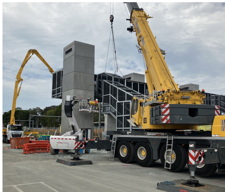
Above: Installation of footbridge staircase to North Road carpark.
